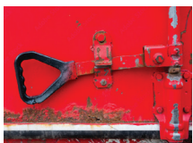
Loose or worn latches
