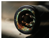
Corroded electrical connectors
